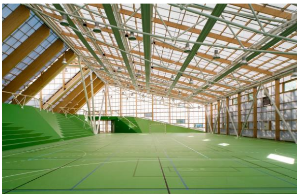
Image 26. Timber and steel used as structural members
