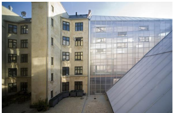
Image 27. Polycarbonate sheets used for facade
