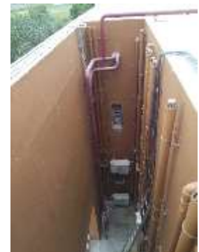
Figure 62 and 63: solar panels and drainage system.
