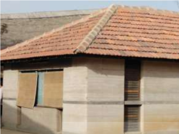
Figure 24: The Mangalore tiles used as a roof cladding.
