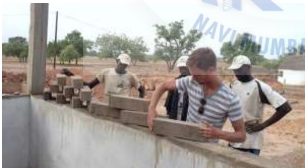
Figure 104: The compressed earth block bricks used for the wall.
