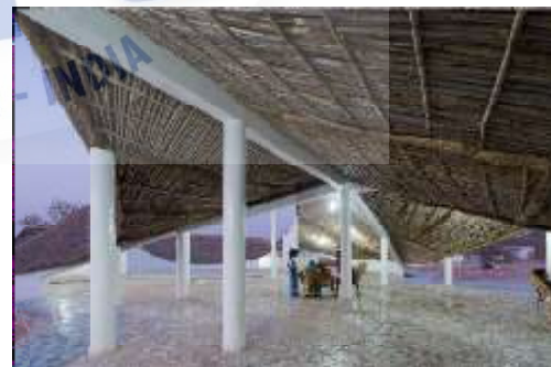
Figure 105: The broken recycled tiles used throughout the structure for the flooring.
