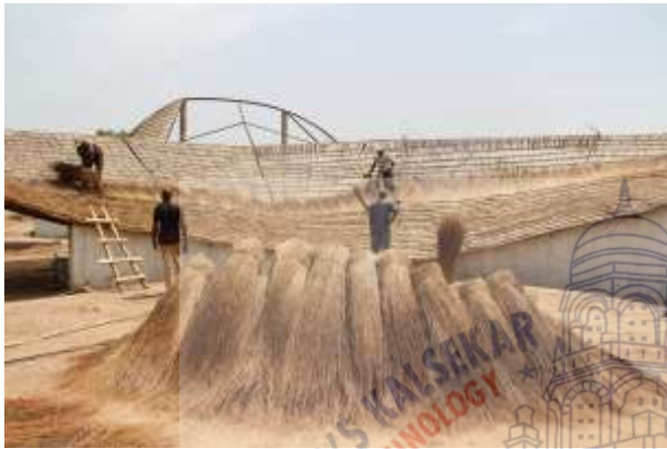
Figure 102 and 103: Bamboo framework and thatch roof
