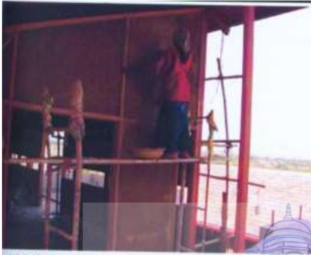
Figure 56: the wattle and daub technique.
