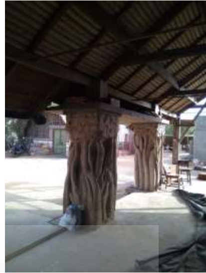
Figure 31: The precast column.
