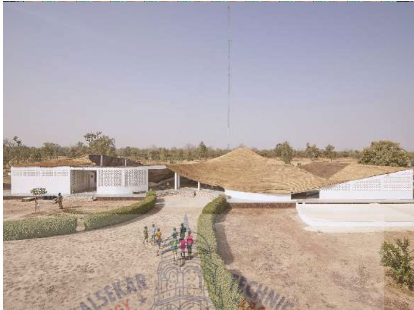
Figure 114: View of the structure
