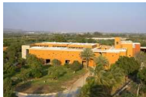
Figure 70: The complete structure
