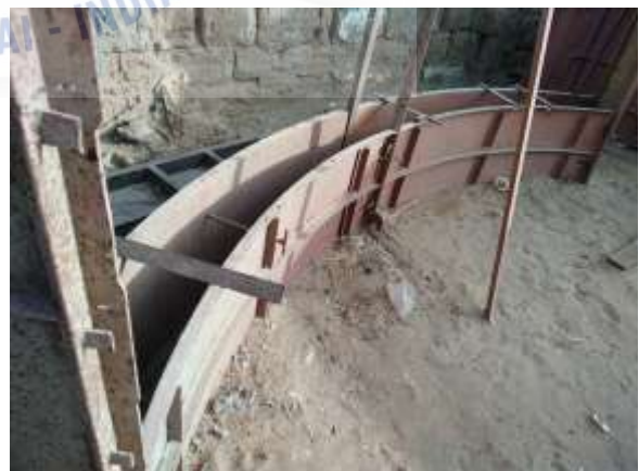
Figure 29: The rammed earth mould
