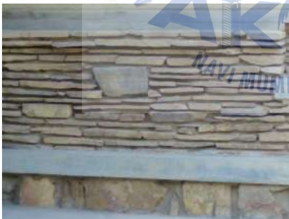
Figure 22: The stone rubble masonry
