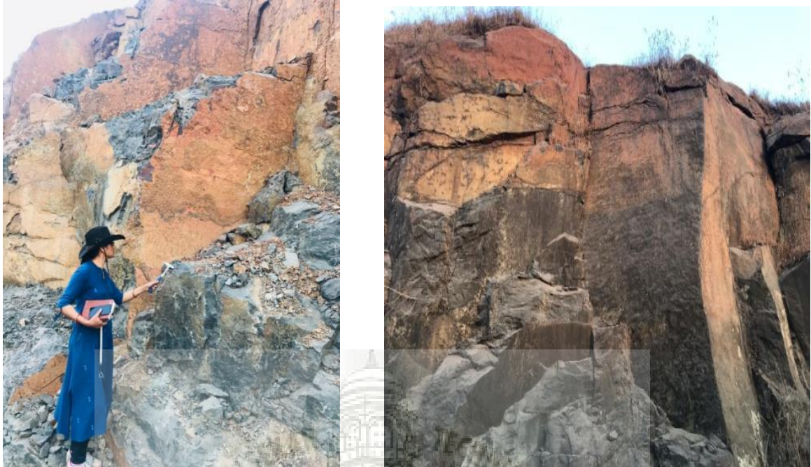
Fig. 3.10 Field photograph showing Weathering/Alteration along Joints
