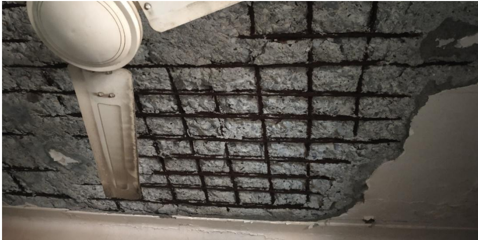
fig no. 5.2 Slab of B-2, Hall
