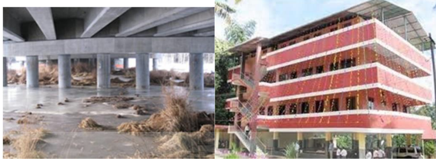
Figure 2.1 Building with open ground storey (1)
