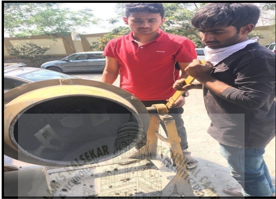
Figure 3.1 Mixing of Pervious Concrete
