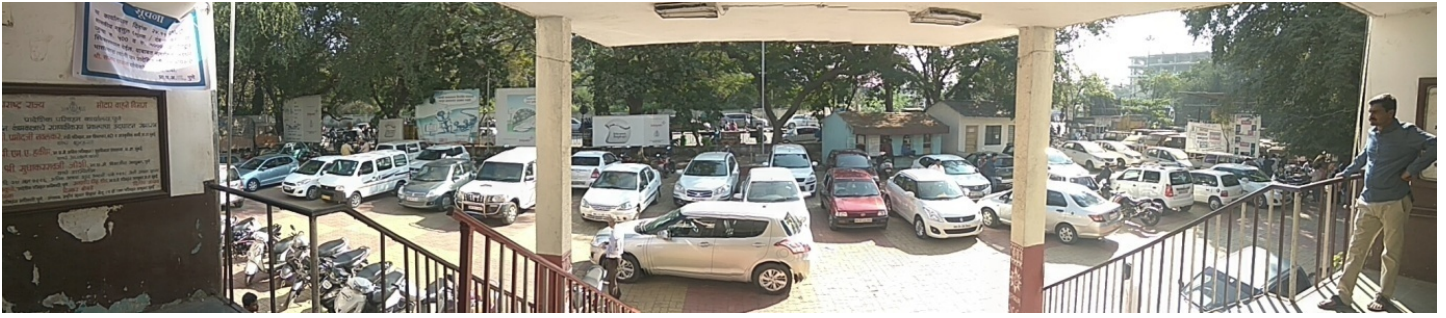
Figure 20 : - Front view of building
