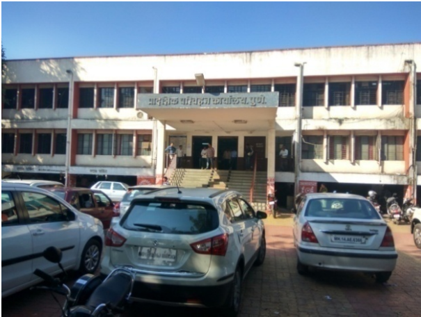
Figure 17 : - Parking in front of building
