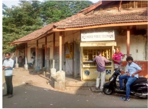
Figure 53 : - Public utility department
