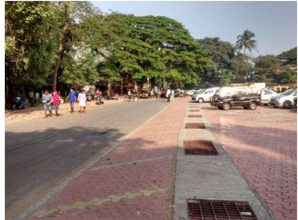
Figure 57 : - Water harvesting system
