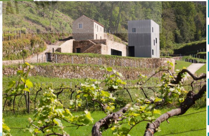
Fig. 4.7.4 shows view of structure from vine yard
