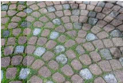
Fig 41: pavement in courtyards
