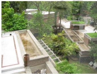
Fig 45: China mosaic tile on roof
