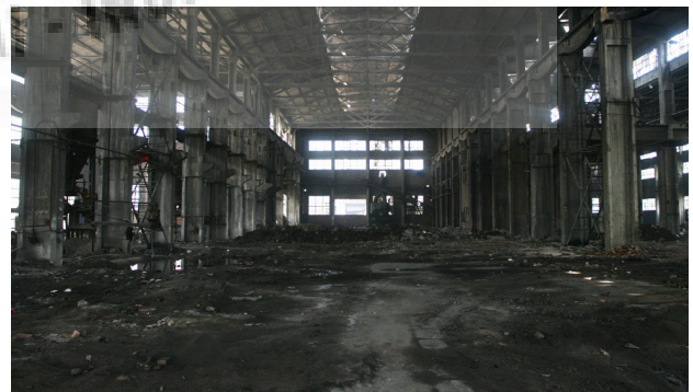
Figure 8.1 -Existing site conditions Hangzhou machine factory
