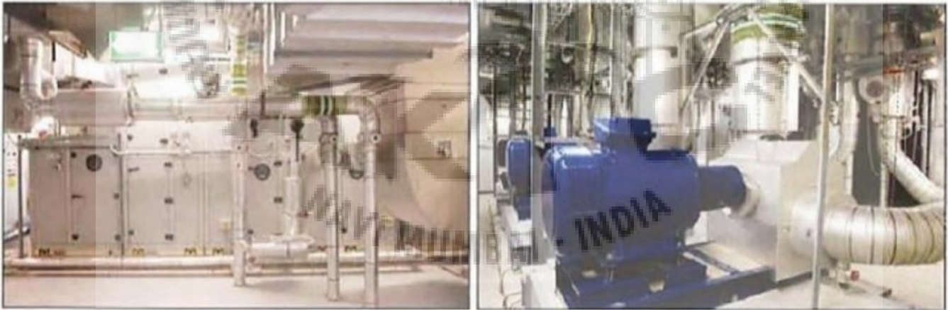
Fig.57. Burj Khalifa Air supply system (Source – archdaily)
