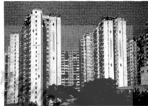
Restrictive Buildings- High Rise buildings Fig. 4
