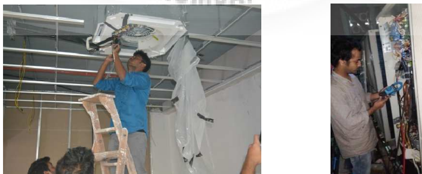
Fig.4.37. Wiring in Indoor and Outdoor unit
