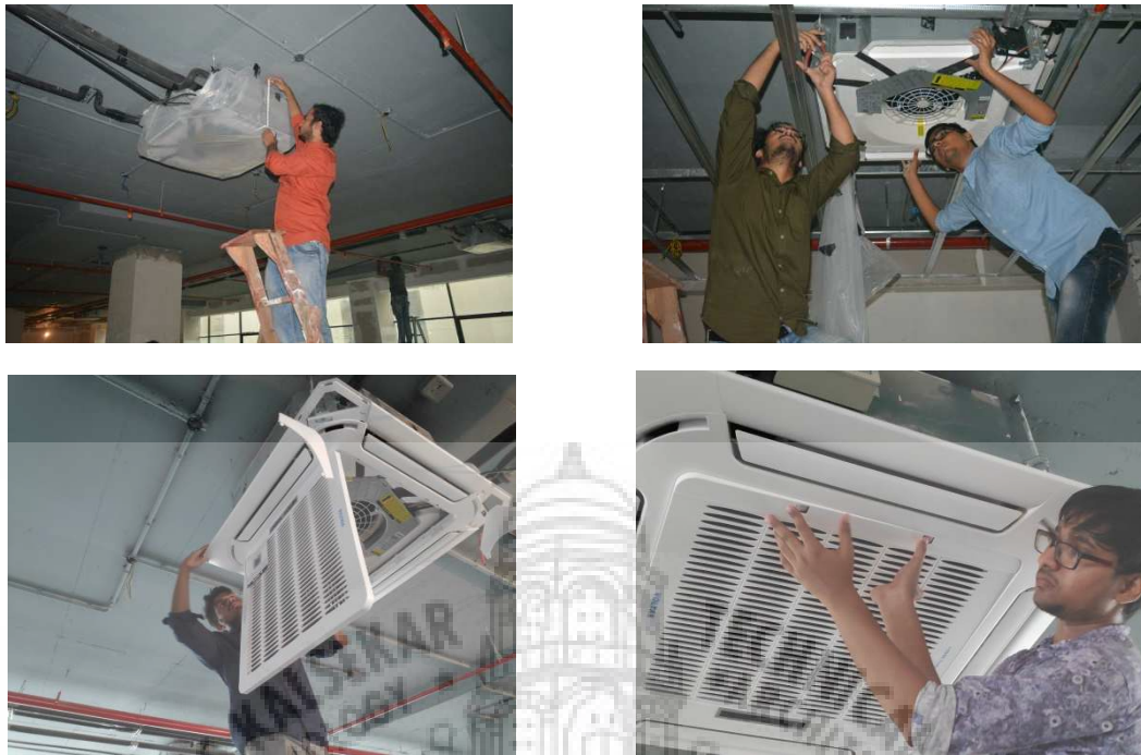
Fig.4.26. Indoor units installation
