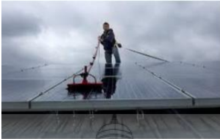
Fig.2.3: Cleaning using vacuum suction
