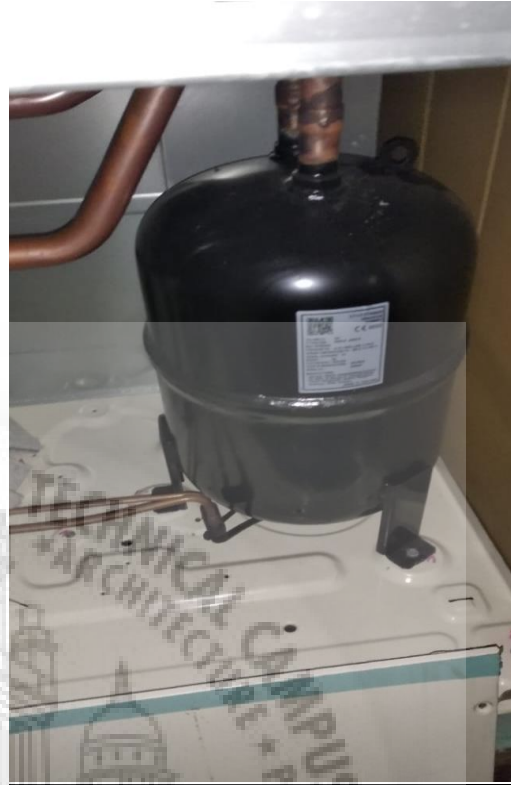
Figure 8-8.Scroll Compressor
