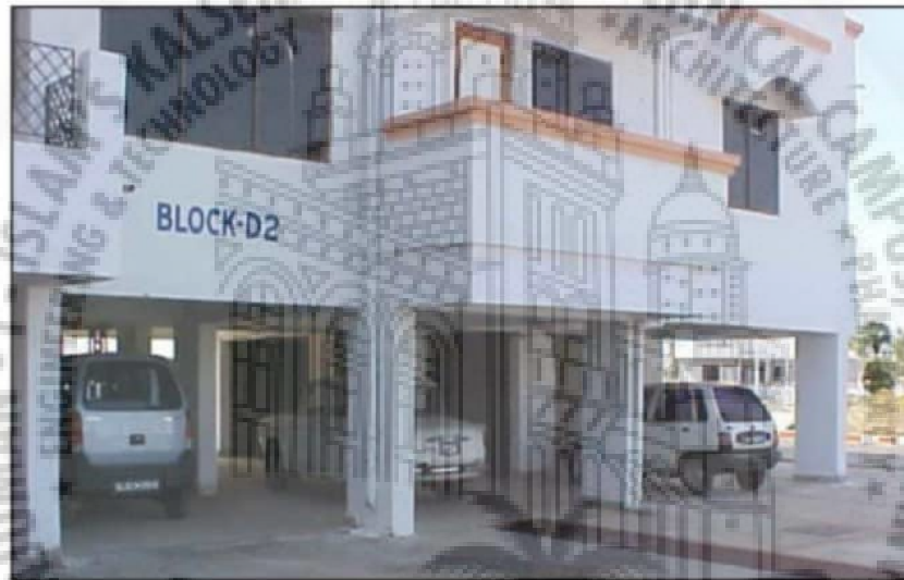
Figure 3.1: Open Ground Storey
