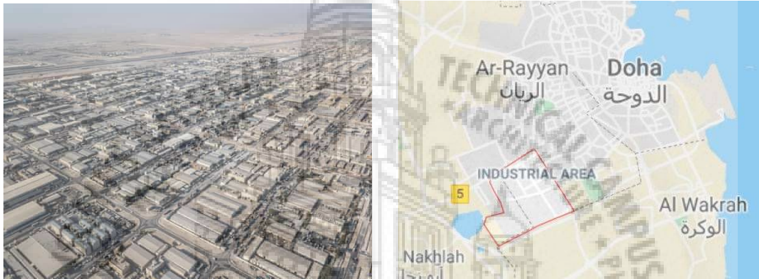
Picture: Overview of Doha Industrial Zone and location on Map
