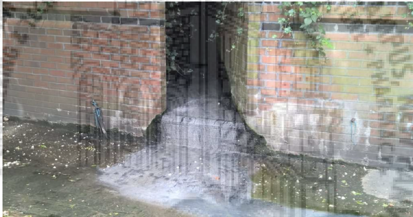
Picture: Wealdstone Brook drain (rooftop and toilet water)
