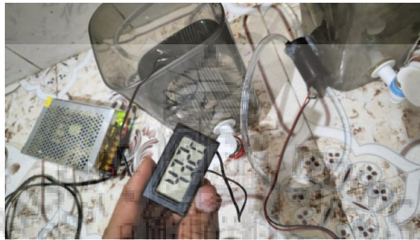
HOT WATER TEMP
