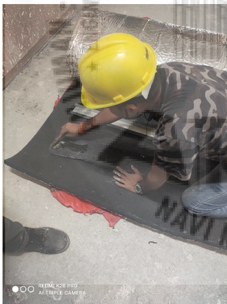
Figure 8-12. Appling insulation & Aluminum tape.
