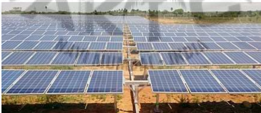
4 MW horizontal single-axis tracker in Vellakoil , Tamil Nadu
