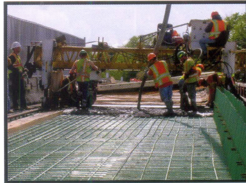
Figure 4: Internally Cured Concrete being Cast at Bartell Road in New York (Wolfe, 2010)
