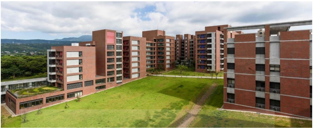
Fig 43. Dormitory Building (MMC )
