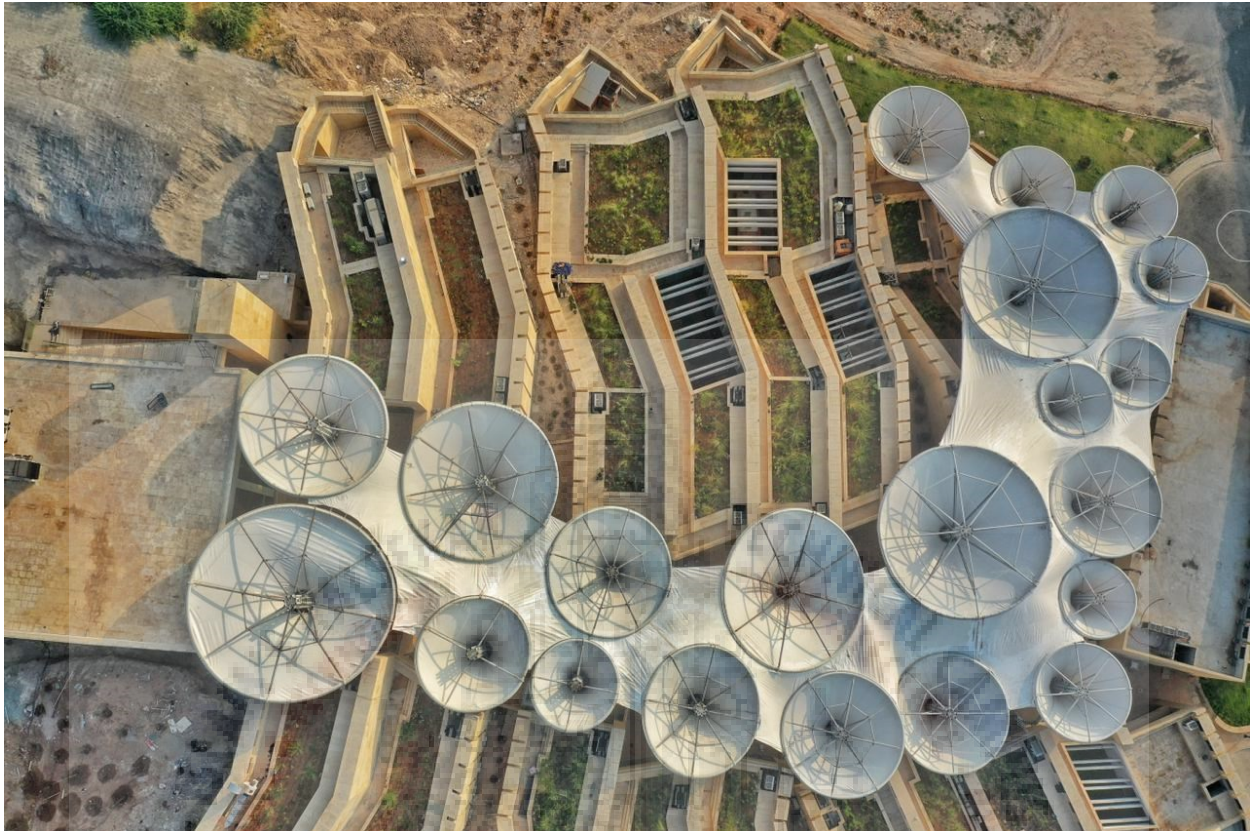
Image 4.14 - TOP VIEW SHOWING TENSILE CANOPY OF THE MUSEUM (Source: ArchDaily)
