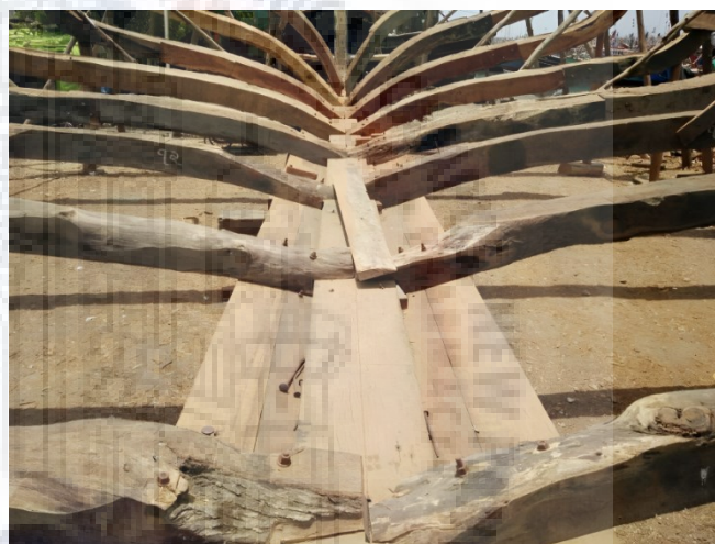
Image 2.2 – Image showing framing of the bridge
