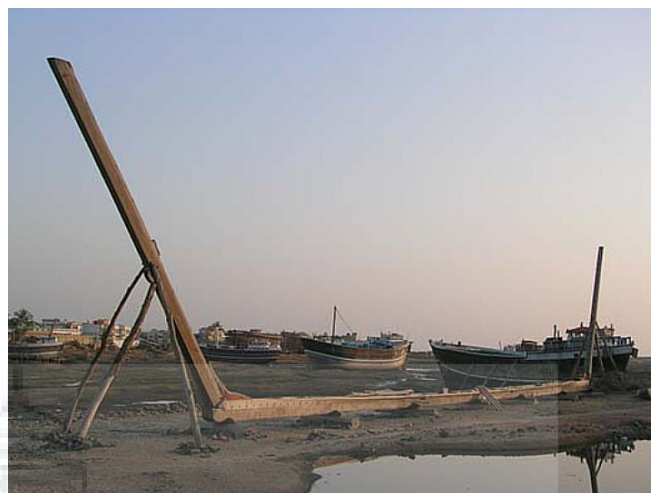
MANDVI SHIPYARD - THE BEGINNINGS OF A SHIP (laying of the Pathan )
