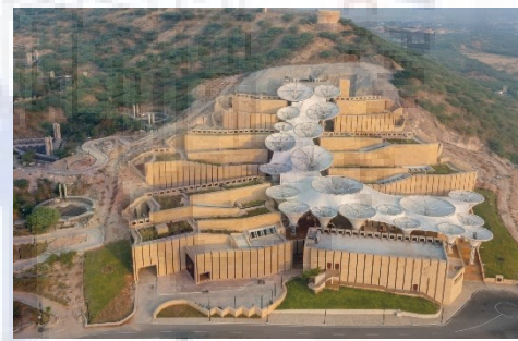
SMRITIVAN EARTHQUAKE MUSEUM, BHUJ
