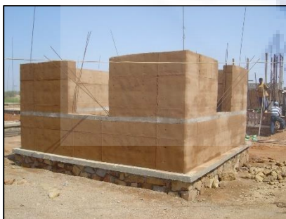
(Figure 56 , construction of earth walls , wattle and daub panels & transition space)
