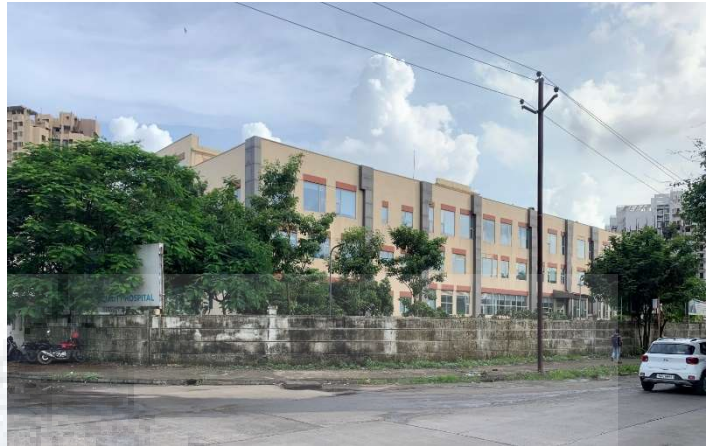
VIEW FROM ADJACENT ROAD
