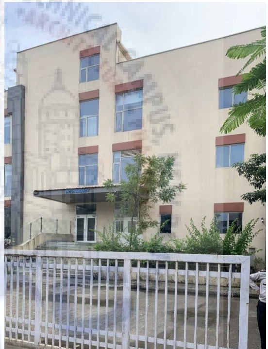
VIEW FROM ADJACENT ROAD
