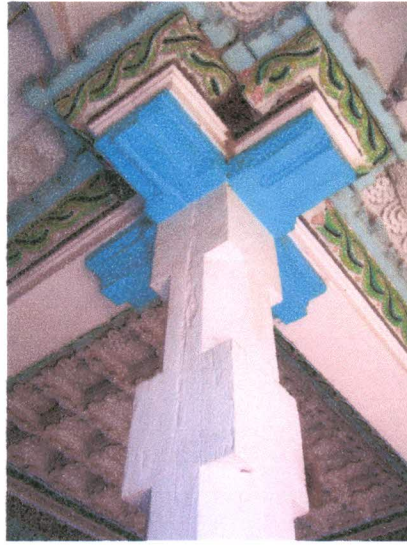
Fig.8 Jamaat Palli: Detail of Column & Ceiling
