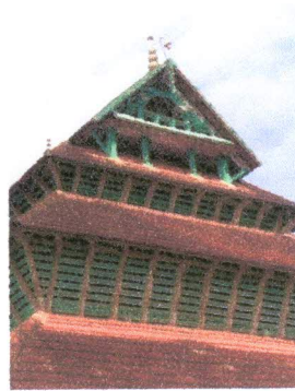
Fig. 5 Mishkaal Palli: Detail of woodwork in gable
