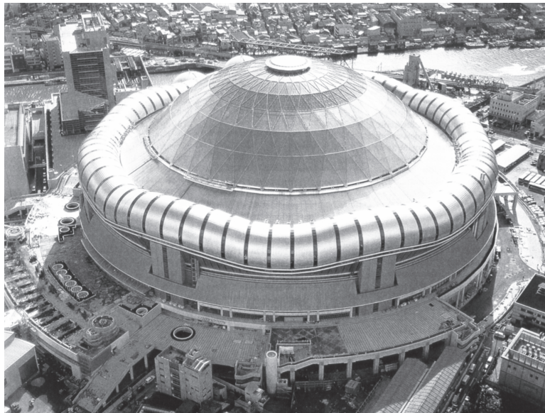
Fig. 15.13 Osaka Dome built in Japan in 1997 ( Courtesy: Steel Today and Tomorrow )
